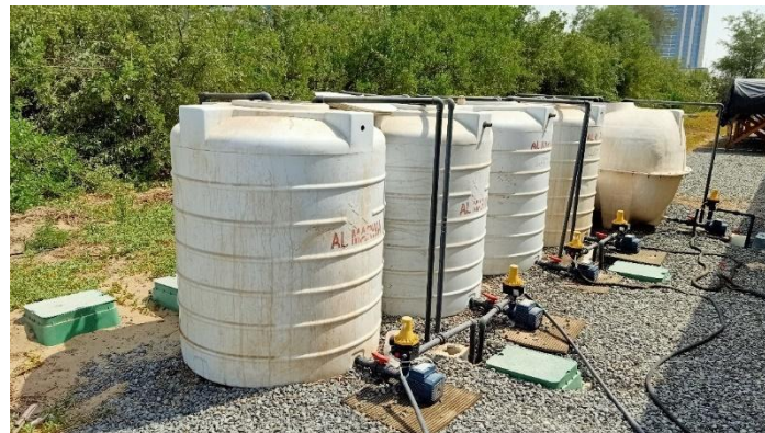
Figure 4. Fertilizer mixing tanks outside the greenhouse.
