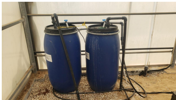
Figure 4. Fertilizer mixing tanks outside the greenhouse.
